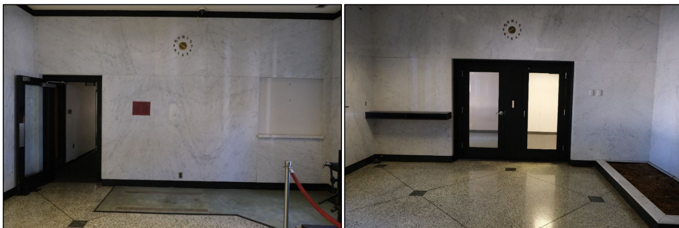
Figure 2. Marble-clad east and west walls, respectively, and terrazzo flooring in the lobby (Image Source: Commonwealth Preservation Group, 2024).
