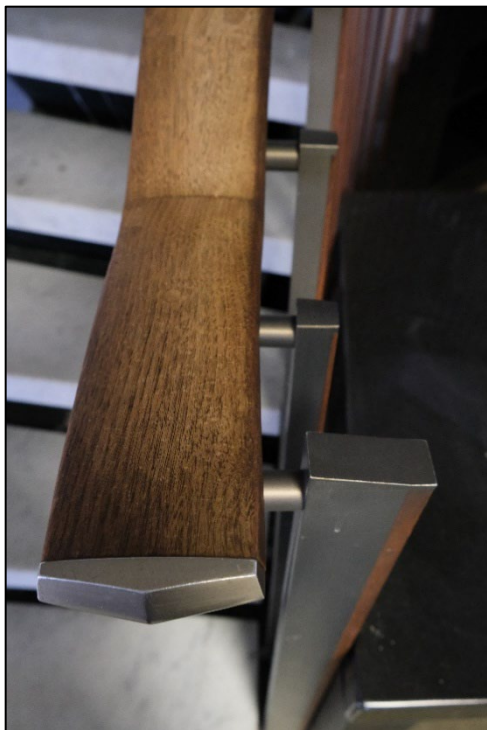
Figure 3. Detail of metal end cap and balusters on stairs (at left) and marble-clad stairs and balustrade (at right, as seen from below) (Image Source: Commonwealth Preservation Group, 2024).
