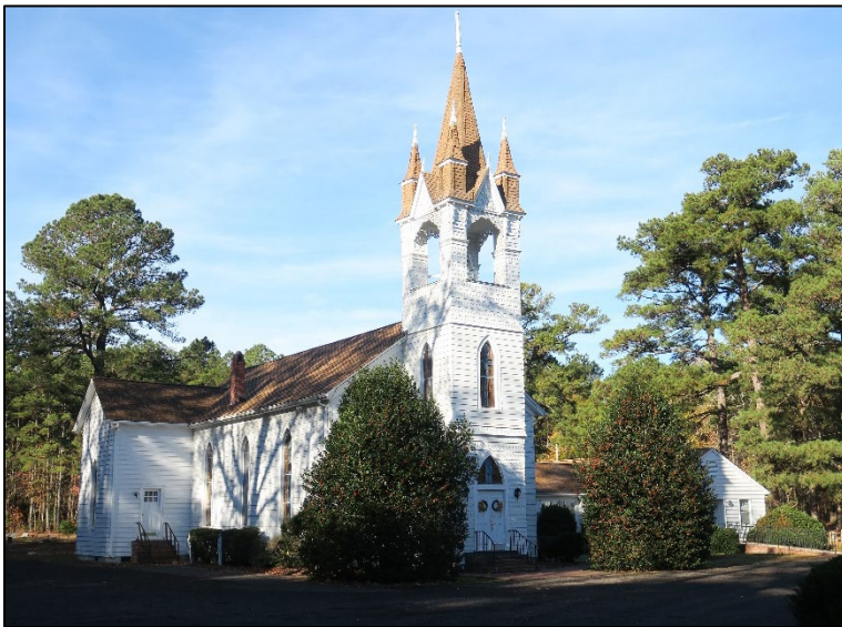
Figure 19. First Baptist Church Mathews (Image Source: Commonwealth Preservation Group, 2024).
