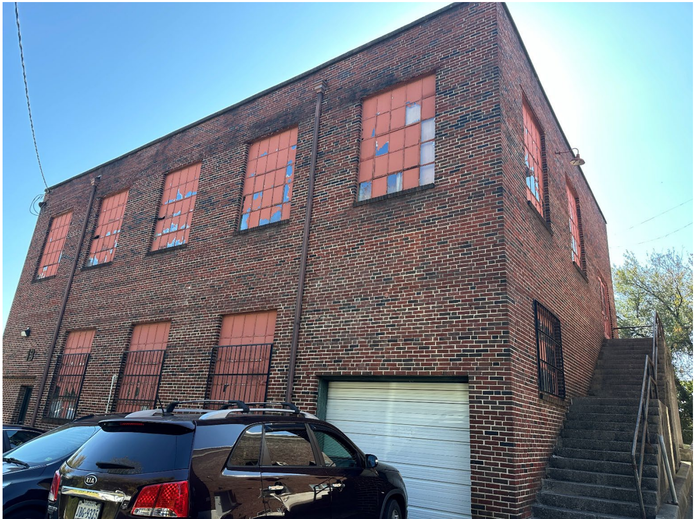
Figure 6 : Front entrance view of the industrial arts annex building prior to demolition, view southeast, October 2024.
