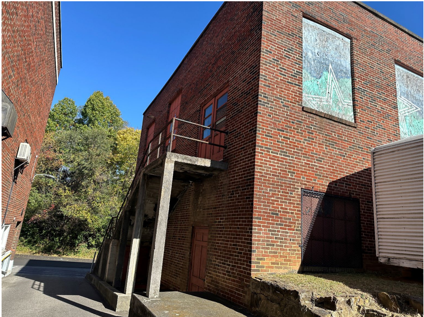
Figure 5 : Small industrial arts annex building to the rear of Lucy Addison High School prior to demolition, view northeast, October 2024. The building served as an industrial arts wing from its construction in the late 1930s until the school's closure as Booker T. Washington Junior High in 1971.
