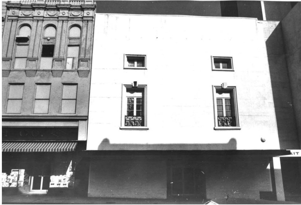
Figure 6: 1980 Architectural Survey Photo of 812 Main Street. Source: VCRIS.
