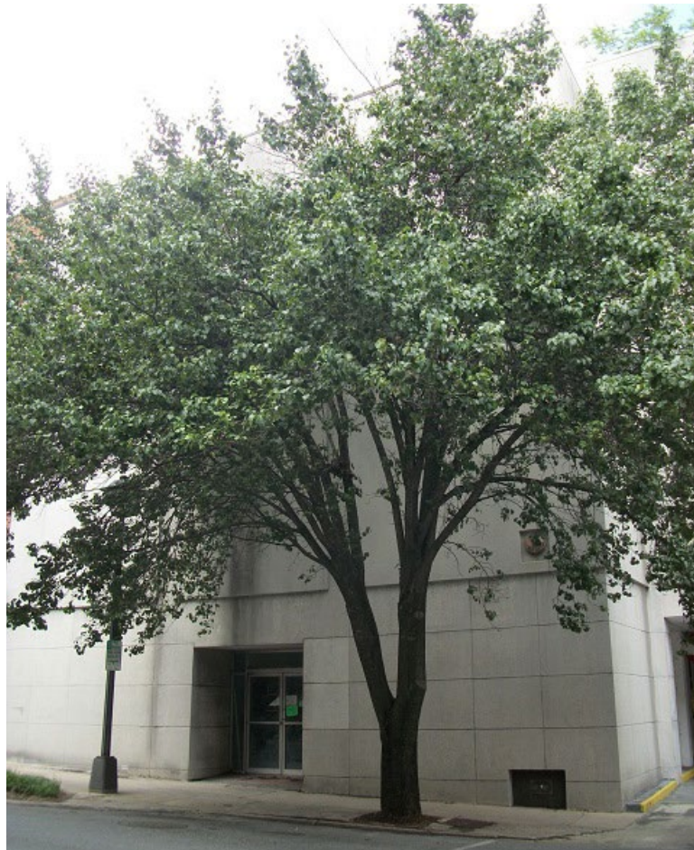
Figure 5: 812 Main Street, 1987 Incompatible Façade Renovation. Source: City of Lynchburg Parcel Viewer
