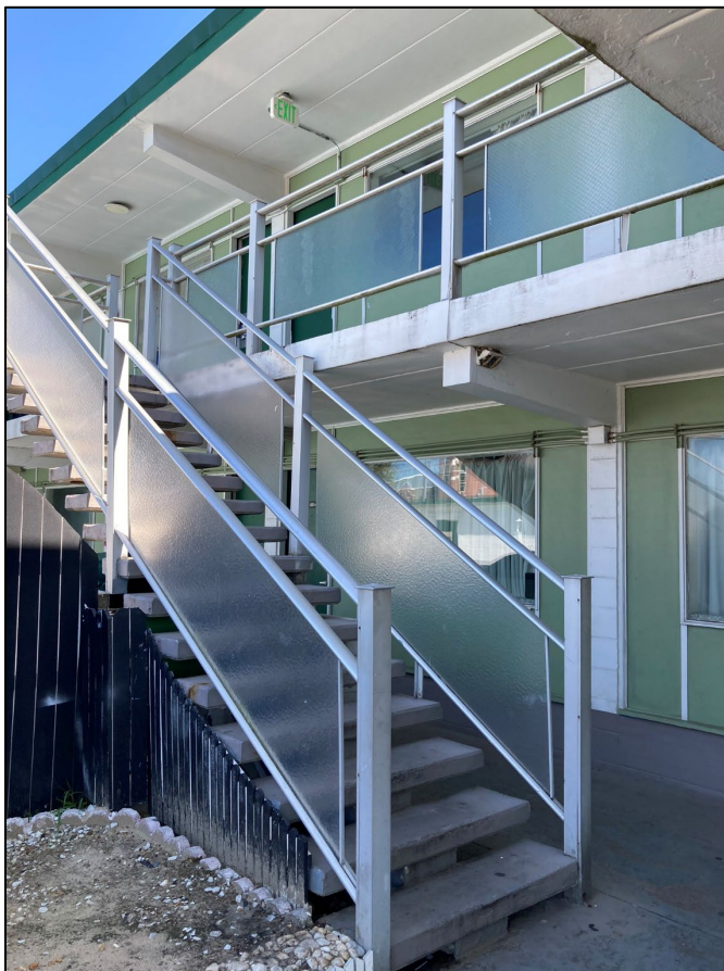
Northern stair and cantilevered balconies at the Beach Carousel. Note the exposed concrete planks visible in the ceiling of the balconies. September 2023.
