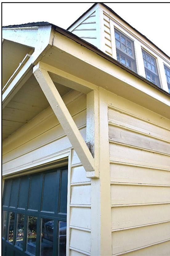
*Figure 12. Garage (ca. 1938), detail of knee brace.*
