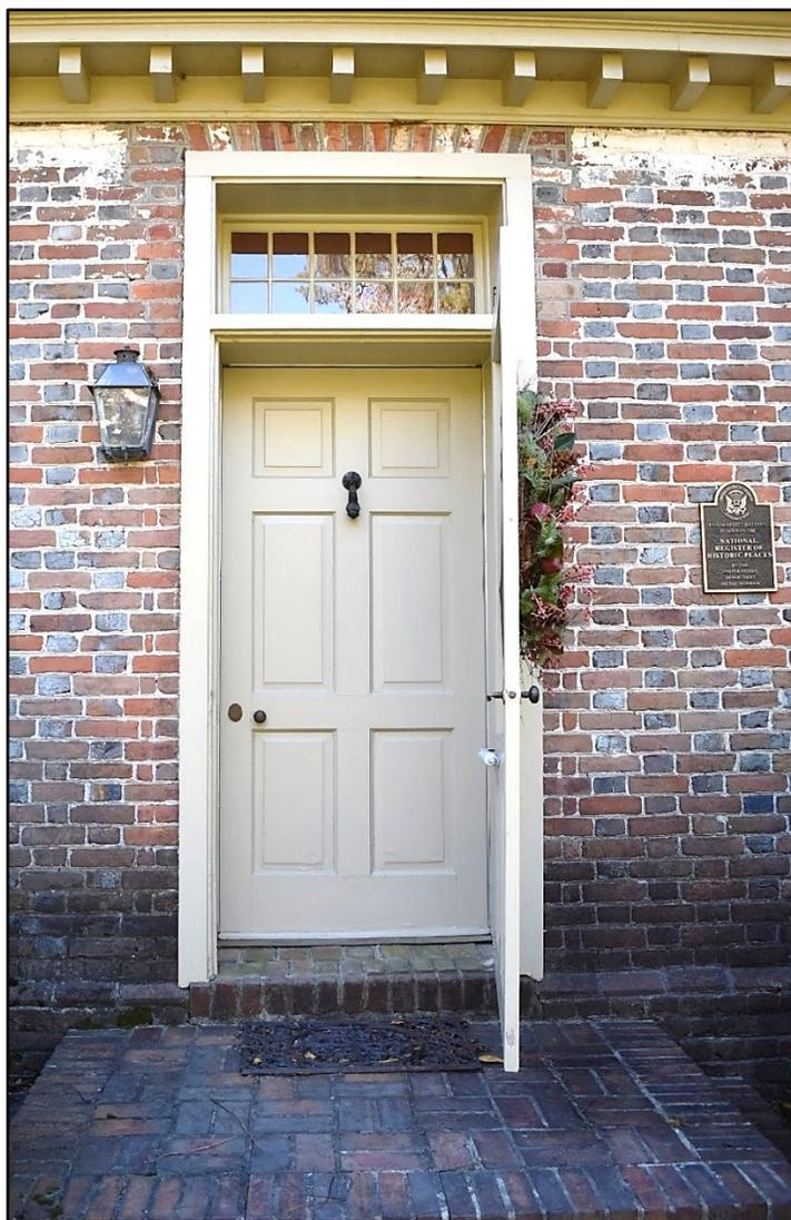
*Figure 4. Detail of east side entrance (replacement door), re-opened transom.
