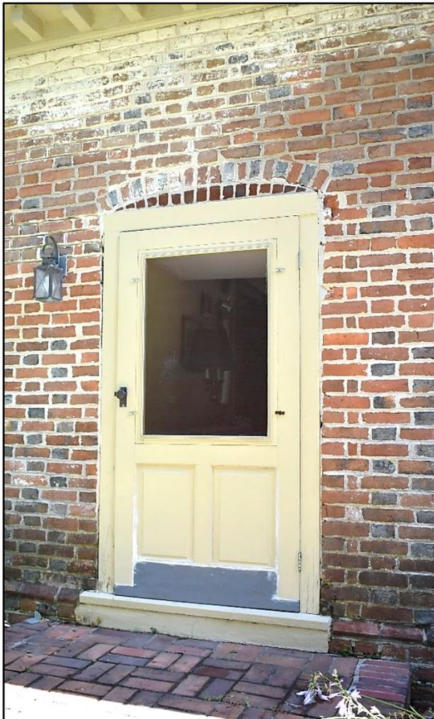
*Figure 3. West entrance door showing alteration to segmental arch.*
