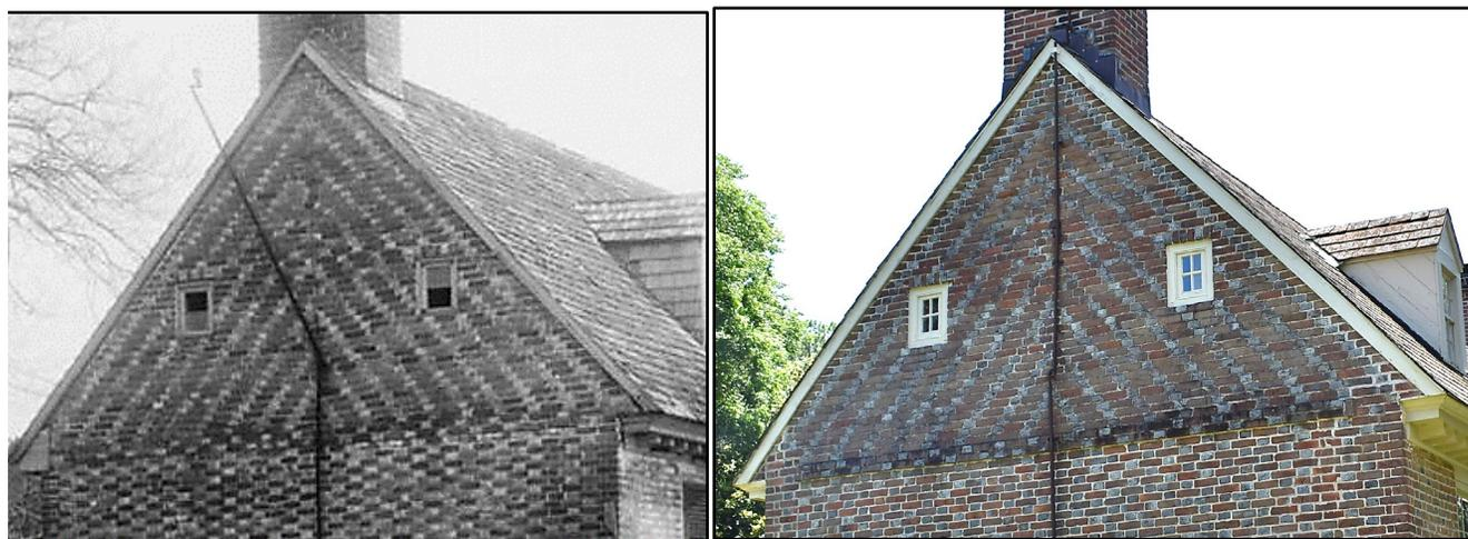
*Figure 13. View of north gable end comparing corner blocks. Left image shows condition in 1934 (HABS), note wooden corner block at northeast eave (left). Right image shows current condition (2024), note that bricks have replaced the wooden block.*
