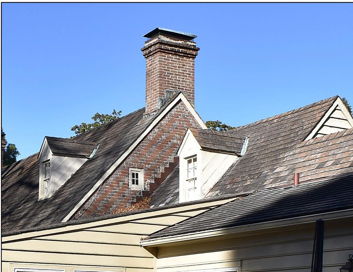
*Figure 5. Detail of south gable end showing glazed header chevron patterning. View to northeast. See Figure 18 for a historical image showing the chevroning pattern.*
