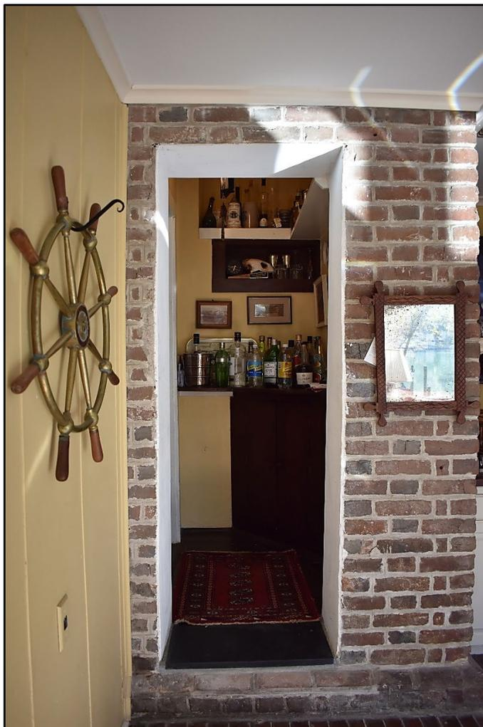
*Figure 11. View from 1950s sunroom into the former dining room closet. The opening was cut into the historic brick wall to allow passage between the addition and the historic dwelling.*
