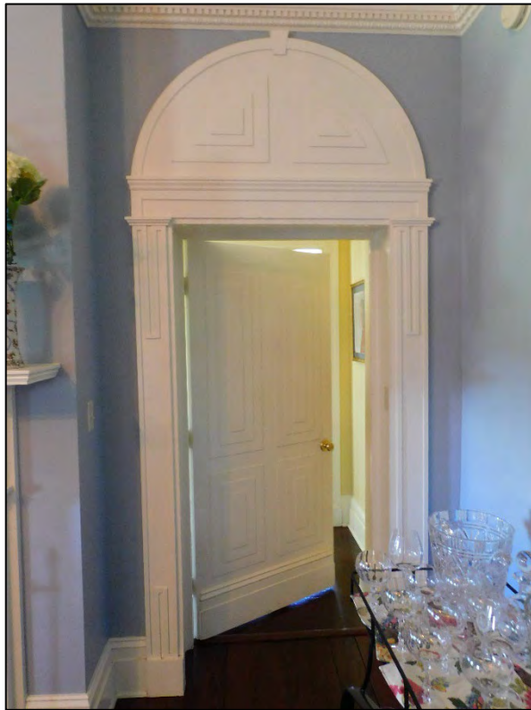
Figure 6: First floor parlor doorway featuring pilasters with a modified Greek key pattern and keyed arch with layered tiered patterns (left). The pilasters are modeled after Plate XXVIII (Figure 4), and the layered tiered patterns are modeled after Plate XLIX in Asher Benjamin's pattern book The Architect, or Practical House Carpenter (1830) (right).
