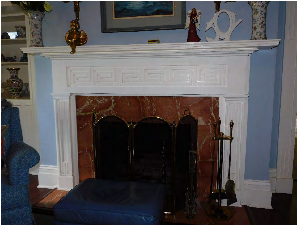
Figure 4: First floor parlor mantel with Greek key pattern on the entablature and pilasters with a modified Greek key pattern.
