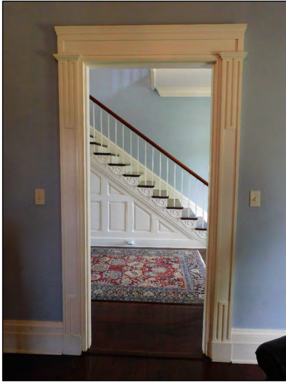
Figure 5: First floor parlor doorway featuring pilasters with a modified Greek key pattern (left), as seen on Plate XXVIII in Asher Benjamin's pattern book The Architect, or Practical House Carpenter (1830) (right).
