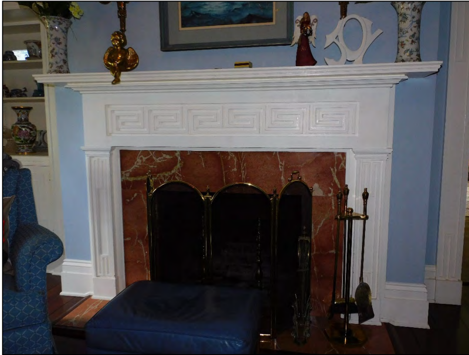
Figure 3: First floor parlor mantel with Greek key pattern on the entablature and pilasters with a modified Greek key pattern.
