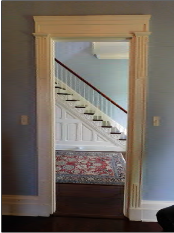
Figure 4: First floor parlor doorway featuring pilasters with a modified Greek key pattern (left), as seen on Plate XXVIII in Asher Benjamin's pattern book The Architect, or Practical House Carpenter (1830) (right).
