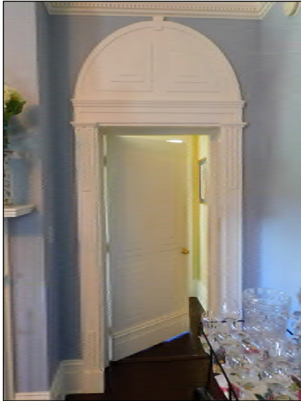
Figure 5: First floor parlor doorway featuring pilasters with a modified Greek key pattern and keyed arch with layered tiered patterns (left). The pilasters are modeled after Plate XXVIII (Figure 4), and the layered tiered patterns are modeled after Plate XLIX in Asher Benjamin's pattern book The Architect, or Practical House Carpenter (1830) (right).
