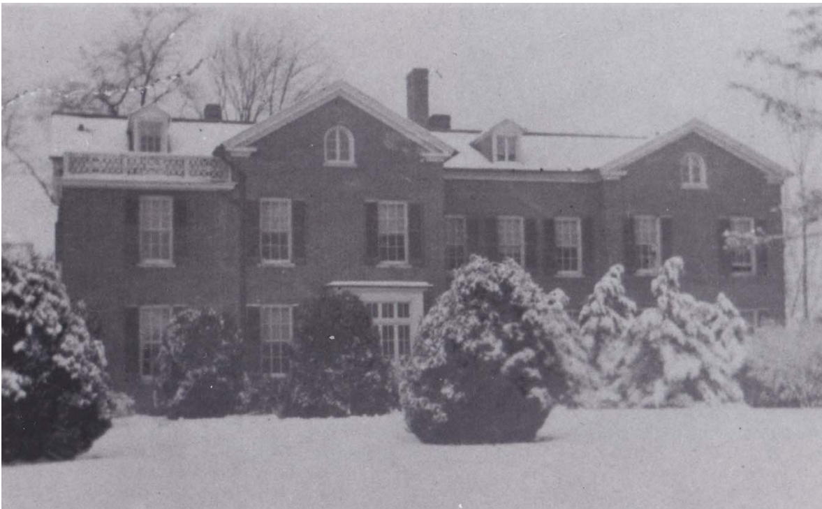
Figure 2: Vint Hill Manor House following the additions and alterations made by Mitchell Harrison, c. 1920. Courtesy of INSCOM and John Salmon.
