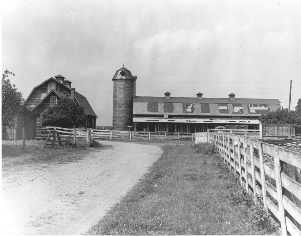
Figure 4: The VHFS Barn Complex prior to renovations by the Army, c. 1942. Courtesy of INSCOM and John Salmon.
