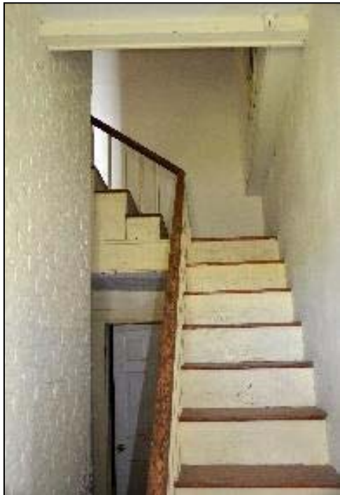
Figure 7. Staircase in the 1865 East Addition.
