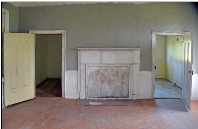
Figure 6. First-Floor Room in East Addition.
