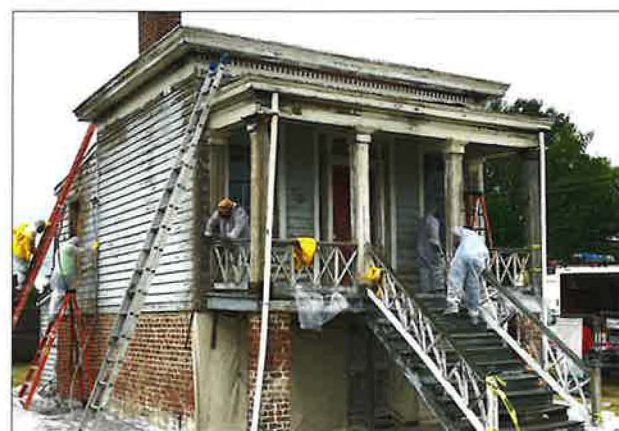
Above: A work crew conducts lead and asbestos removal.
