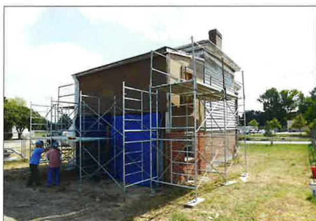
Above: A work crew conducts lead and asbestos removal.
