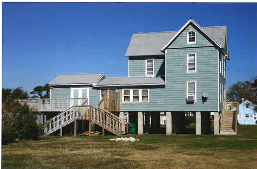
Some property owners are already taking measures to protect their historic homes from rising sea level. In the town of Saxis, several buildings have been lifted on concrete block or wooden piers.
