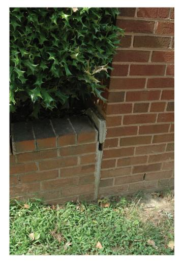
Figure 44. Planter has rolled away from west face of 1976 addition.
