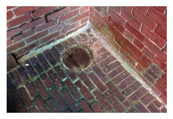
Figure 30. Pointing at deck of north porch – 1939 wing.
