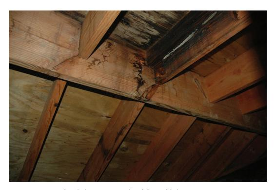
Figure 53. Damage from leaking at eastern edge of flat roof deck.
