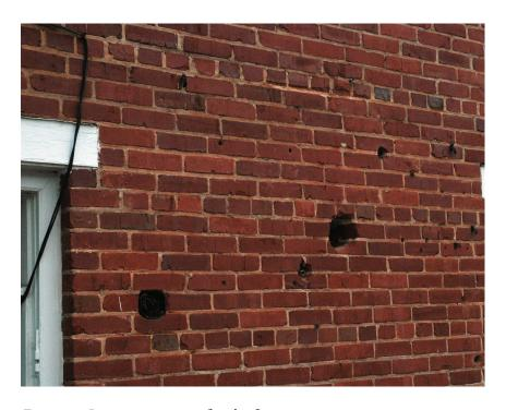
Figure 37. Penetrations in east facade of 1939 wing.
