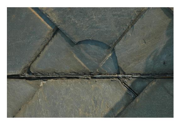
Figure 14. Closed valley of slate roof.
