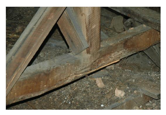
Figure 48. Sagging girder below northeast corner of the cupola.
