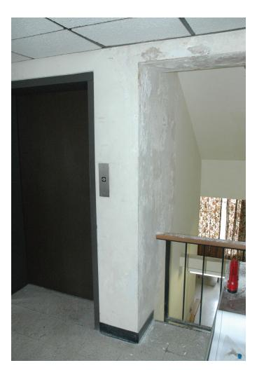
Figure 56. Damaged plaster at the elevator shaft.
