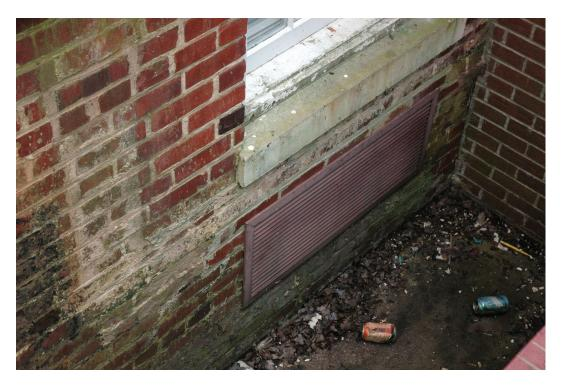
Figure 34. Ghost of former window well in north areaway.
