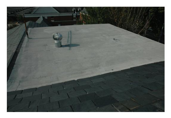
Figure 15. Asphalt roofing on flat deck.
