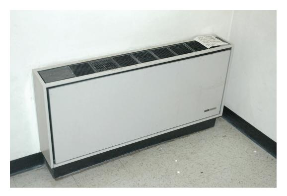
Figure 58. Typical fan coil unit.
