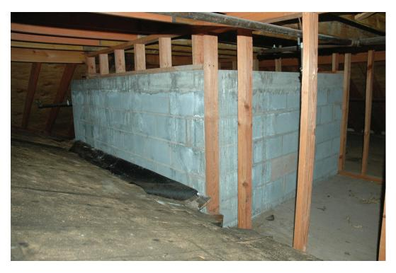
Figure 54. Evidence of water running down sides of elevator shaft.
