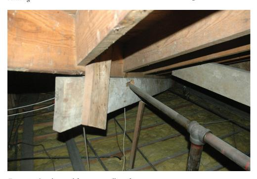
Figure 51. Supplemental framing at valley rafters – 1939 attic.
