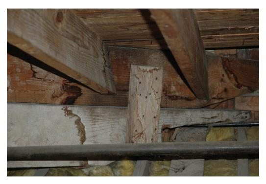
Figure 52. Evidence of roof leak – 1939 attic.
